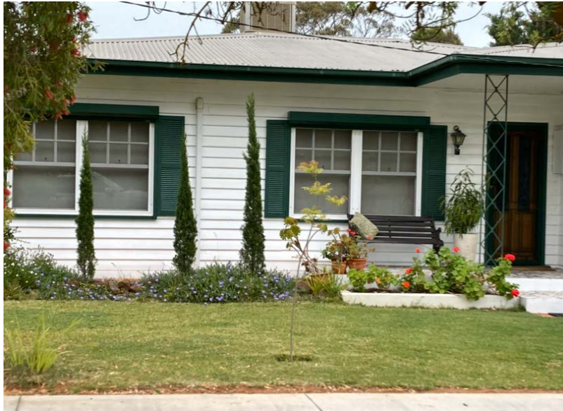
Weatherboard House in Kaniva
