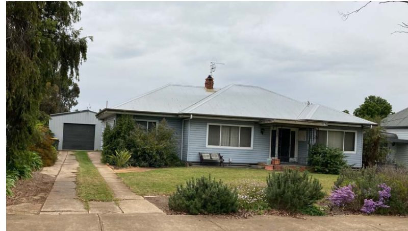
Weatherboard House in Kaniva
