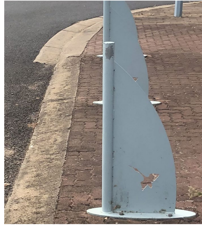
Existing bench seats and bollards to be relocated (where required) and refurbished including repainting in new colour (i.e. colourbond 'Ocean Blue') and replacement of timber slats
