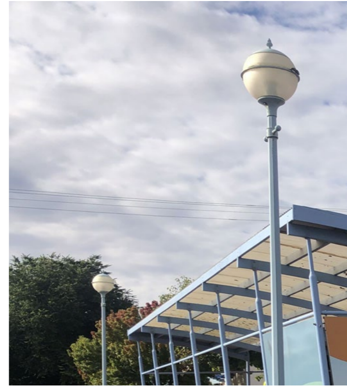
Existing lights - repaint in new colour to compliment Edenhope's marketing / branding strategy (ie. Colorbond 'Ocean Blue')
