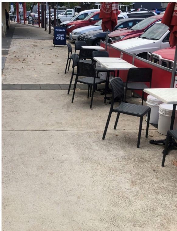
Standard concrete paving with tool joints in a grid pattern
