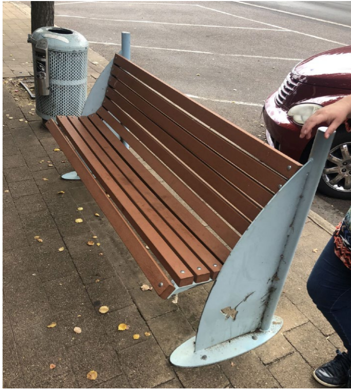
Existing bench seats and bollards to be relocated (where required) and refurbished including repainting in new colour (i.e. colourbond 'Ocean Blue') and replacement of timber slats
