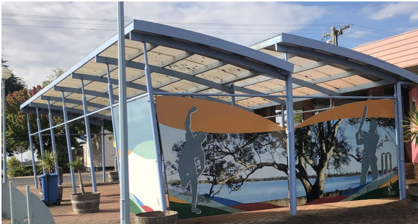
Renovate (replace roof sheeting) and re-paint existing shelter in new colour
