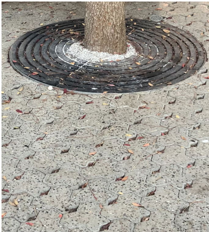
Permeable paving to surround existing / proposed street trees with cast iron / steel tree grate.
