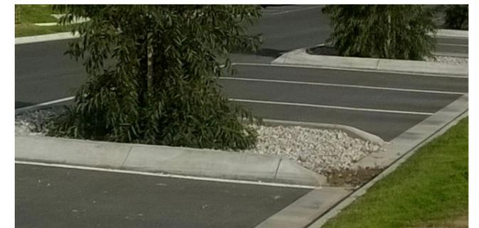
Kerb modifications to provide passive irrigation to tree bays and median strips
