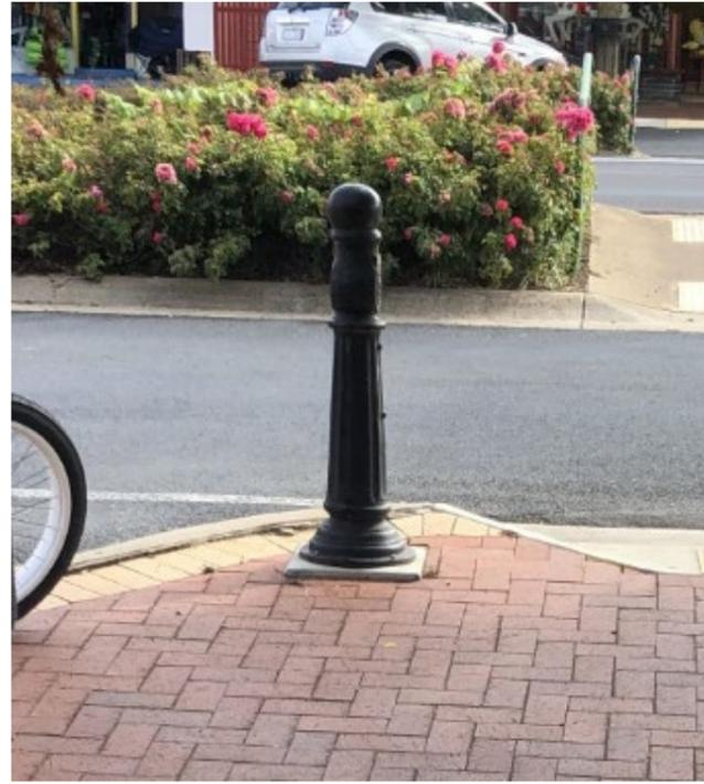
Existing cast iron bollards to be repainted and relocated. Some new bollards required with chain link barrier between.
