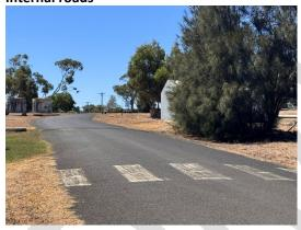
The roadway leading into the reserve from Budjik Street is sealed. There is a speed hump located fairly close to the entrance with a 10km per hour sign located next to it. The zebra crossing needs repainting.
