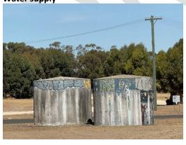
The water supply at the reserve was updated recently. This has enables more efficient and cost-effective watering of the existing playing surfaces and enables opportunities for additional playing surfaces to be constructed and maintained. Water tanks are located behind the Sporting Complex, next to the Community Hub. The fire service tank holds 120k litres. There is also a bore that services the site. It provides 500 litres per minute free flow and has an 18kw submersible pump.
