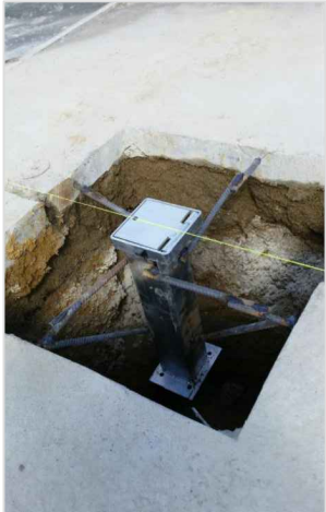
TYPICAL DETAIL FOR SLEEVE INSTALLATION - CUT OUT METHOD FOR CONCRETE PAVEMENT
